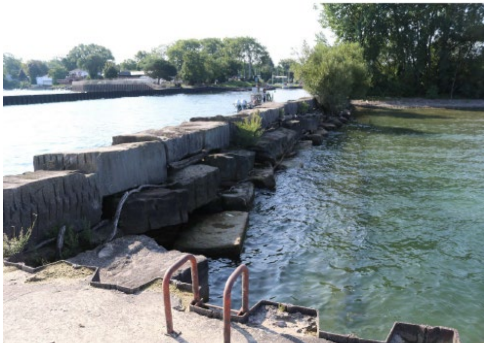
Figure 3: Wilson West Pier Reach B.
