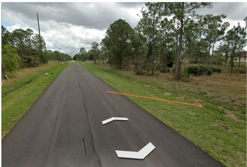
Figure 3 Looking west along the road at the project site. Arrow identifies road side swale the extends from the review area to the east and west.
