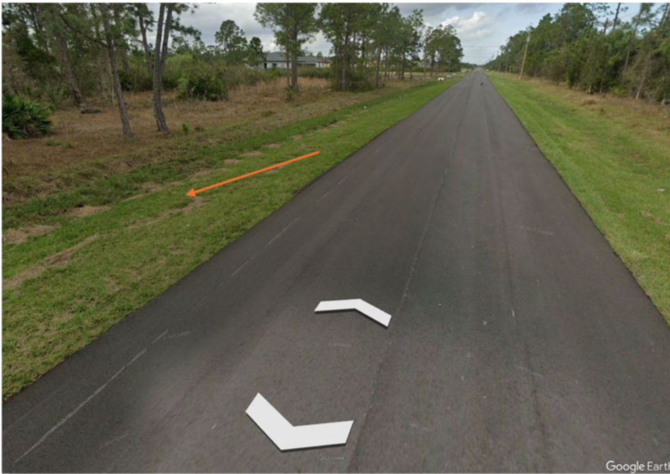
Figure 2 Looking east along the road at the project site. Arrow identifies road side swale the extends from the review area to the east and west.
