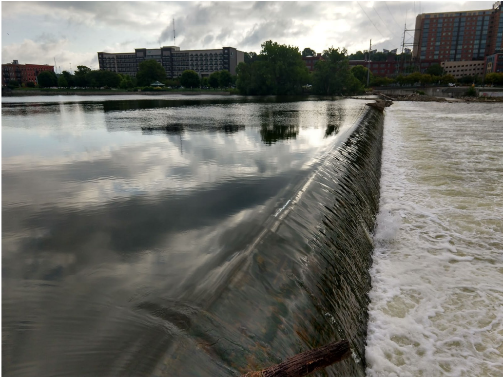
Existing 6 th Street Dam (fixed crest)
