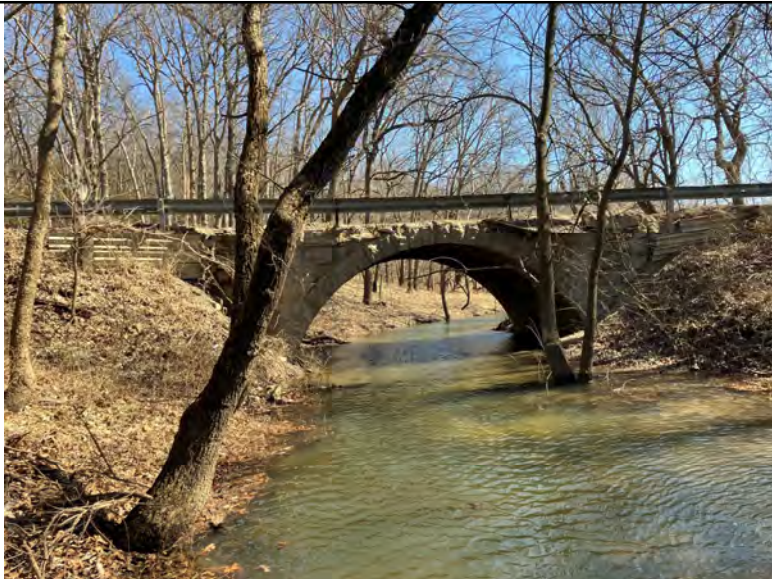
West Elevation View
